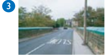
View across Victoria Bridge out of Conservation Area.
