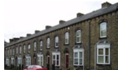
Figure 25 & 26: Nos 12-24 Hopwood Street share an unusual feature of a sloping roofline following the incline of the street. Properties on the opposite side of the road share a more typical stepped roofline as the street slopes down towards its junction with Huddersfield Road
