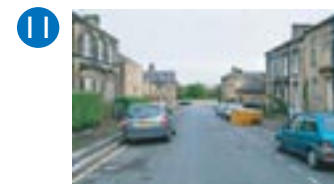
View out of Conservation Area from Hopwood St.
