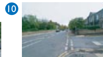
View into Conservation Area along Huddersfield Rd.
